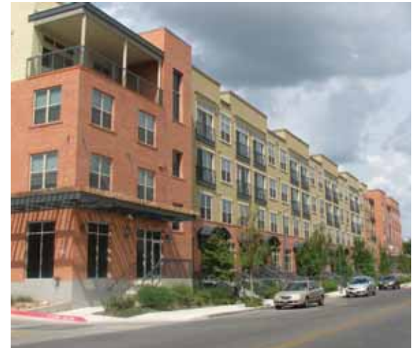
Providing a variety of housing choices in walkable and bikeable neighborhoods located near transit, employment, retail, medical and recreational amenities is part of the housing vision.
