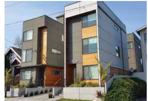
Stacked flats in Seattle, Washington integrate four well-designed residences into a standard single-family parcel.
